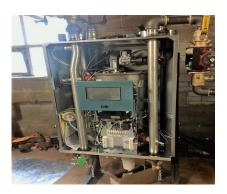
Here is a picture of the inside of one of our two new furnaces. They are high efficiency (which means we should save on gas costs), modulating boilers (which means that they can adjust the heat output dynamically, resulting in more even heat delivery to the building). They do not look anything like our old boilers: there is a lot of high tech in them.
